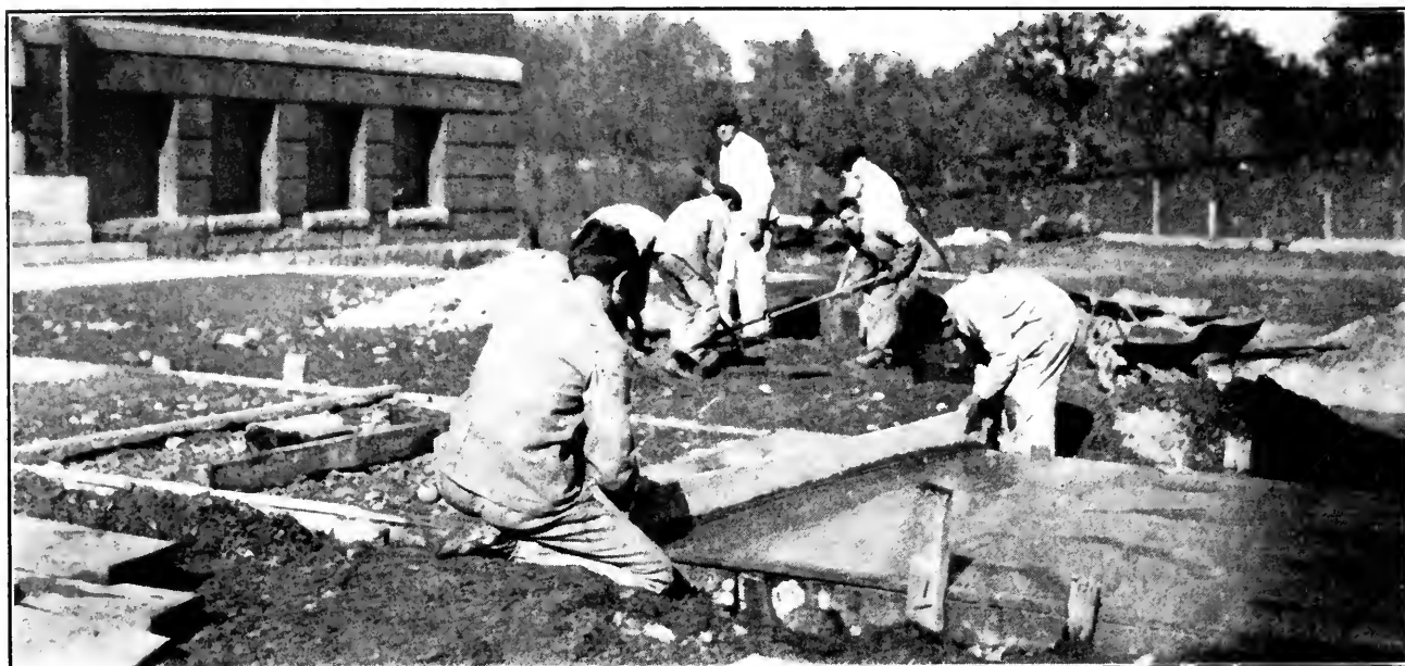
A CLASS IN CONCRETE WORK
